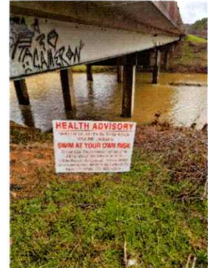
Site 4 Signage placed 3/4/25
