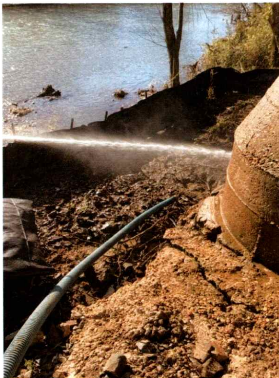
MH 1748 During cleanup
